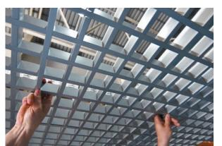
A small gap between the cassette and the T-profile is allowed at the cross T-profile joints, because the profiles
